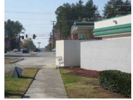
Figure 4.12: LOW SCORE: Large blank walls are negative features next to the sidewalk, such as this wall along Hwy 54 in Durham.
